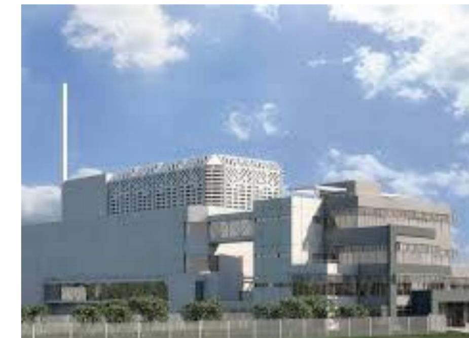
RA10 2015 (under construction)
